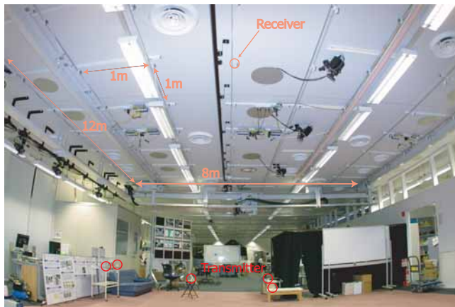
Fig.6 Experimental system consisting of 88 receivers embedded on ceiling
